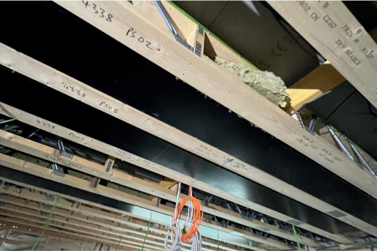
Figure 4. Panels in metal web type joists
