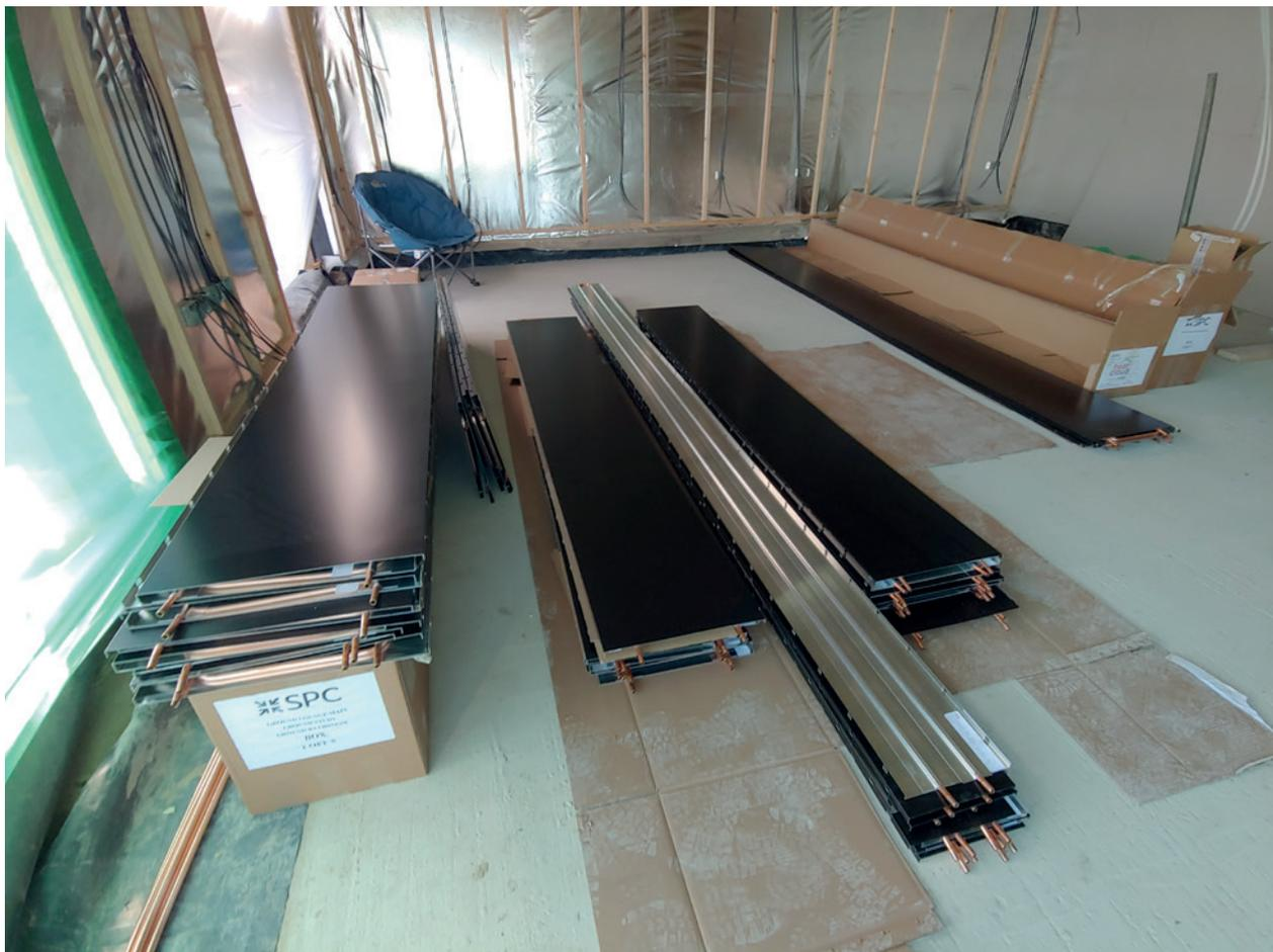
Figure 1. Heat Cloud panels being unpacked
