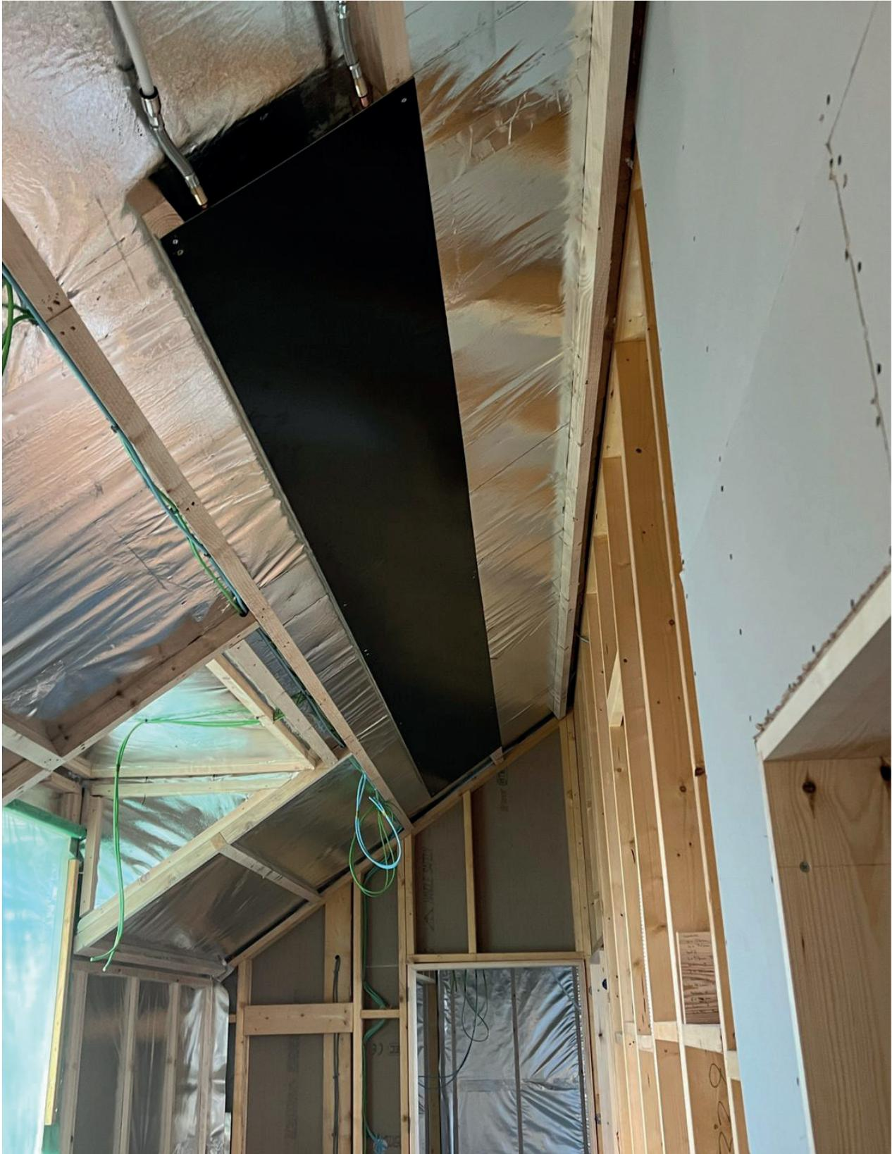
Figure 4. Panels in metal web type joists
